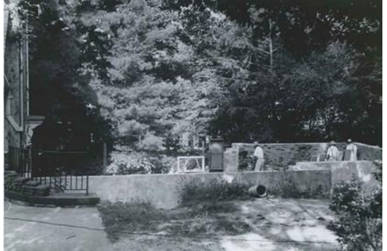
Garage Basement Construction, 1967. A3.48
