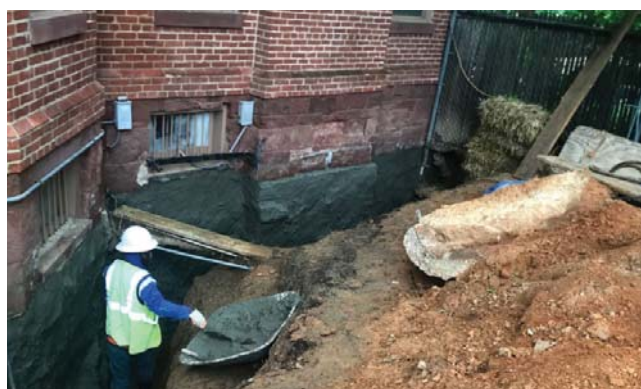
Federal Masonry Restoration contractors completed the stabilization and waterproofing of the foundation of the Dower House in June.
